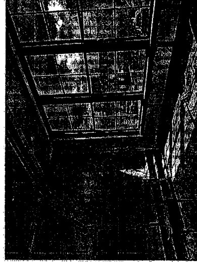
Figure 9 Existing large window bays and mullions
